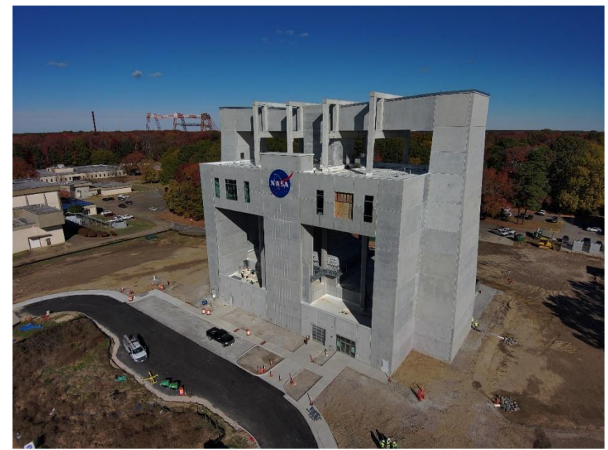
FDRF construction progress (Nov. 22, 2024)
