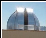
JPL Ground Terminal Table Mtn, CA
