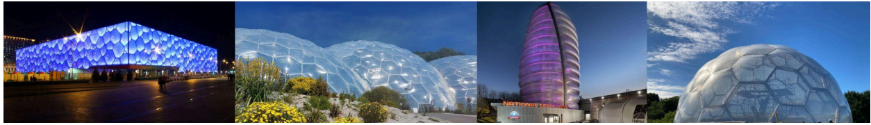
Figure 47. Examples of ETFE "pillows". From left to right: National Aquatics Building, Beijing 2008, The Eden Project Cornwall, England, 2000, The National Space Centre Belgrave, UK, 2001, Cleveland Metroparks Zoo Rainforest Dome, Cleveland, OH
