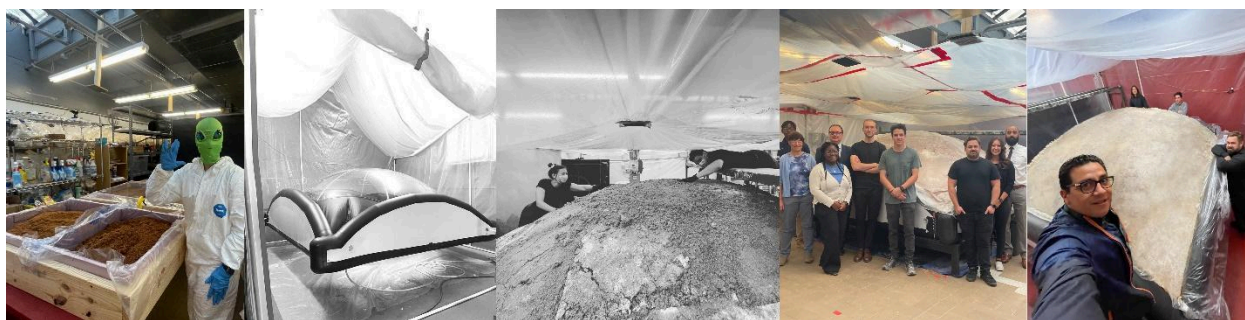
Figure 4. Photos of living prototype production. From left to right: “Alien” making mycopanels, inflated dome form before panels are placed, placing the living material on the dome, NIAC mid-review as the mycelium dome had freshly started growing, full mycelium dome weeks after mid-review.
