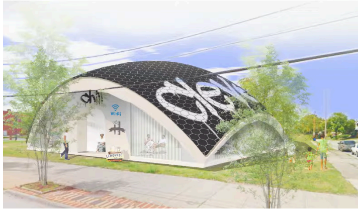
Figure 58. Concept for THE CHILL. A biodegradable bio-insulation is made in between reusable inflatable layers to make temporary cooling stations in urban centers for people at risk of heat related illnesses or death. The inflatable-mycomaterial concept was directly derived from this NIAC study.
