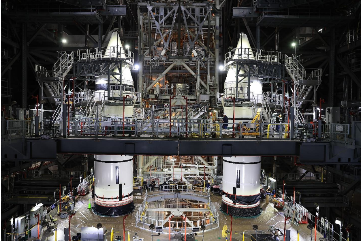
Fig. 3 Artemis II solid rocket boosters completed stacking February 19.
