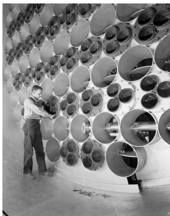
(a) View looking upstream. GRC-1958-C-47803.
