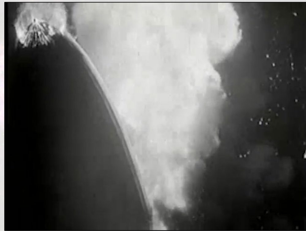
Subsequent Firebrand Hazard (doped fabric and painted girders)
