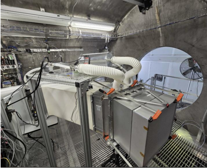
Figure 3. Pleated Filter Testbed Configuration at MSFC with the TCC Tray attached. Showing basic test article installation.
