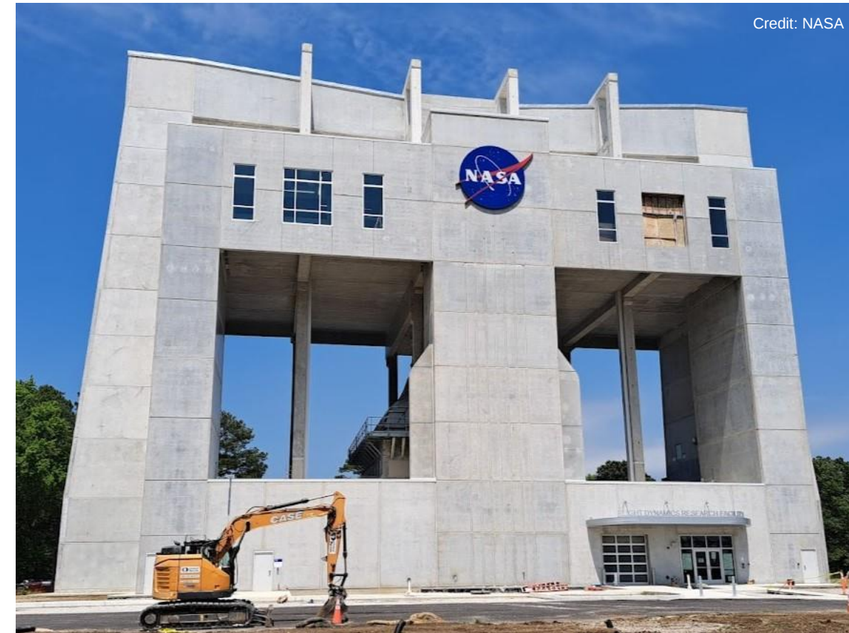
FDRF construction progress (May 14, 2025)
