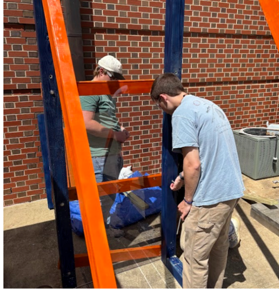
Figure 7-2: Initial Wall Assembly w/o Attachments
