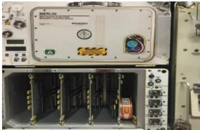
Galley (Water, PWD, Food Warmer) Crewed vehicle may be different
