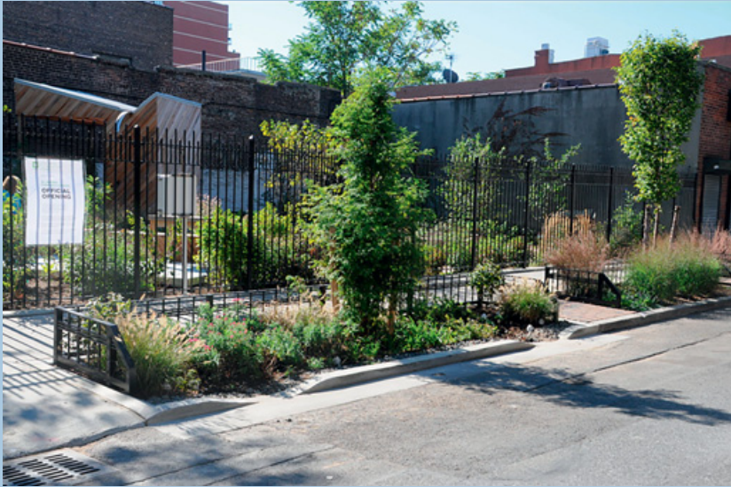
Figure 21 Rain garden installations at Denton Place, Brooklyn, New York City, part of the Green Infrastructure Plan. (Source: Kohler, 2023)
