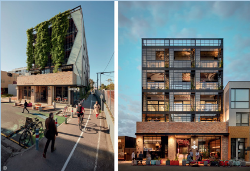
Figure 8 Left: The Commons, Melbourne, with increased bike lanes, open frontage, and green wall (Source: Tom Ross, 2013). Right: The façade of Nightingale 1, made of recycled brick. (Source: Peter Clarke, 2017).
