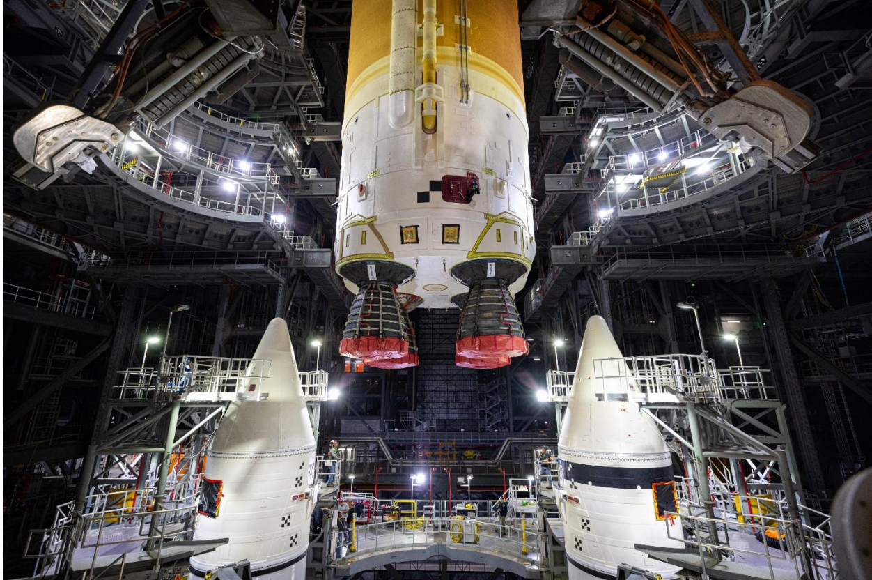
Figure 4: The SLS core stage for Artemis II was mated with the solid rocket boosters on mobile launcher 1 in March 2025.
