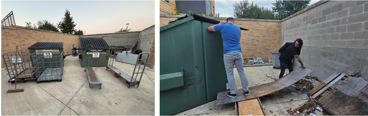
Fig. 32 Progress of site transformation on the UT San Antonio campus.
