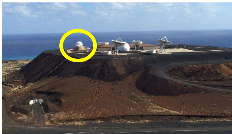
Figure 3. Image of Cottar Hill on Ascension Island showing the CIF (large central building), weather tower (left in yellow circle), James Benbrook facility (right, foreground steel tower in yellow circle), and ES-MCAT facility (right background building in yellow circle).
