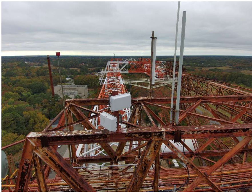
Figure 2: GA-9120 Panels Installed on Langley Gantry
