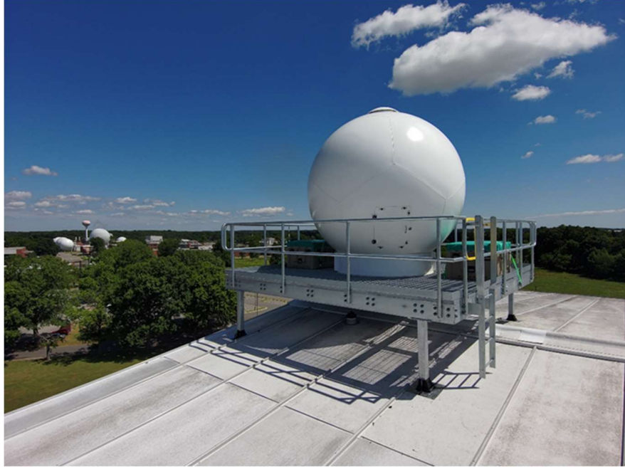
Figure 1: LSTAR Installation on NASA Langley Research Center Hangar
