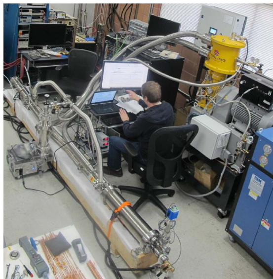
Fig. 237.—A turnkey He-gas-cooled CORC ® cable with CT-to-RT terminations. The terminations are currently a large portion of the system mass and will require weight reduction for aerospace applications (Ref. 237).
