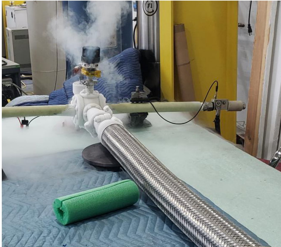
Fig. 249.—Prototype cable demonstration system commissioning during ampacity testing.
