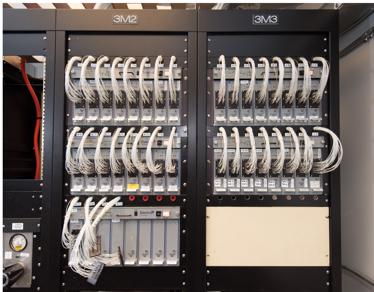
Figure 38.—NetScanner™ pressure scanning system.
