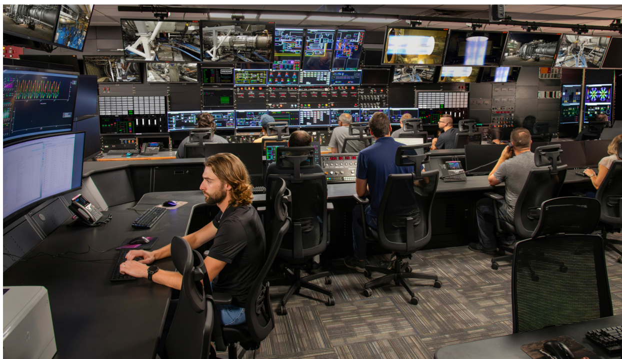
Figure 10.—PSL control room. (GRC-2025-C-07467)
