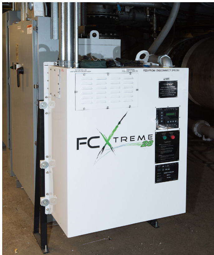
Figure 24.—PSL 28-VDC engine-starter power. (C-2014-08197)
