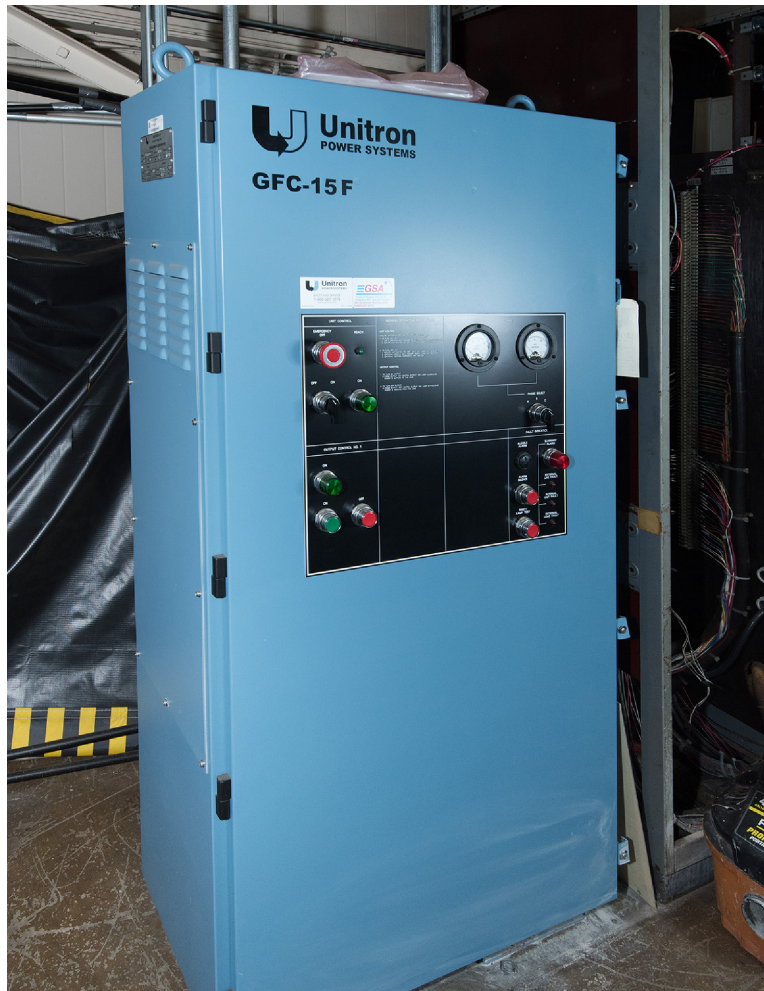
Figure 25.—PSL 400-Hz power supply.
