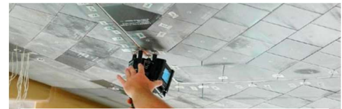
Tile Gap Inspection
