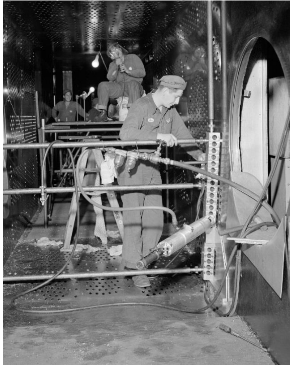
C-1956-42930 Porosity hole drilling operation in 8x6 SWT, 1956
