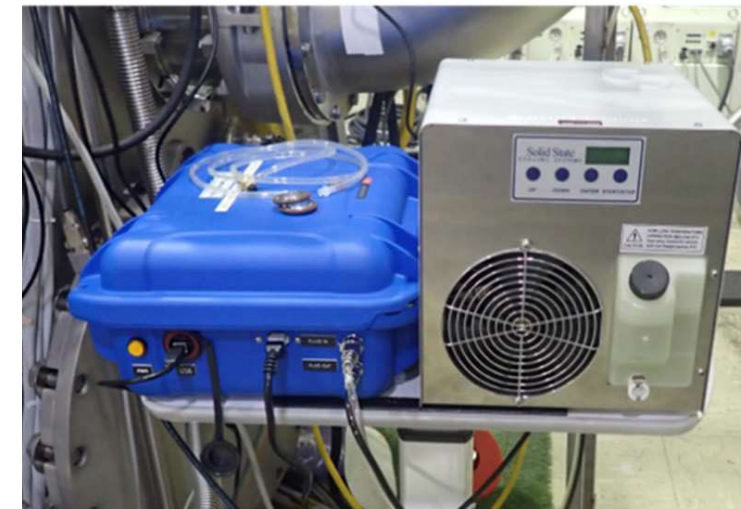
Control Box & “Chiller”
