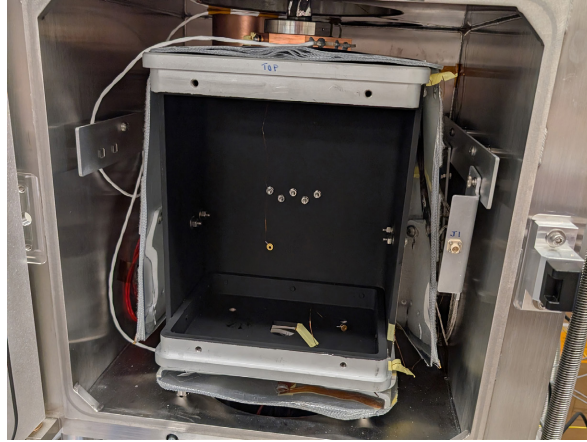
Figure 8. LESTR Unit 01 cold box.
