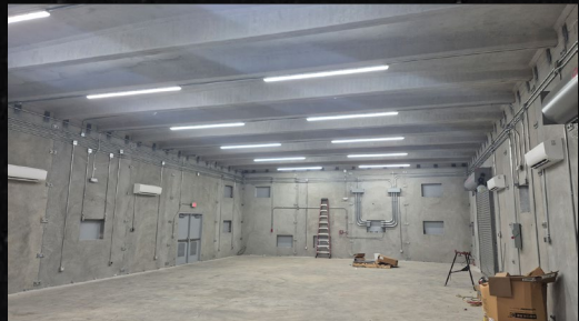
Facility 2: Potential cryogenic/high- pressure refueling facility (JSC)
