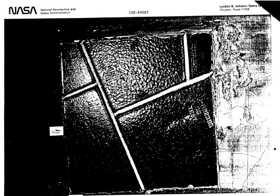
Exceeding temperature capability of tile leads to bubbling of RCG coating and shrinkage of tile substrate.
