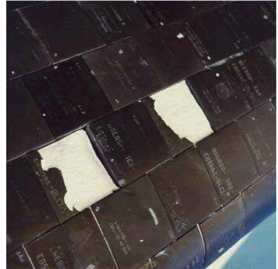
Loss of tiles on STS-2 due to lack of waterproofing
