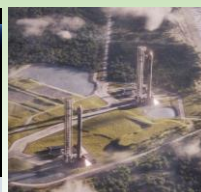
2nd Pad at Cape (LC37) Complete
