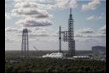
Blue Origin LC-36B Rebuild
