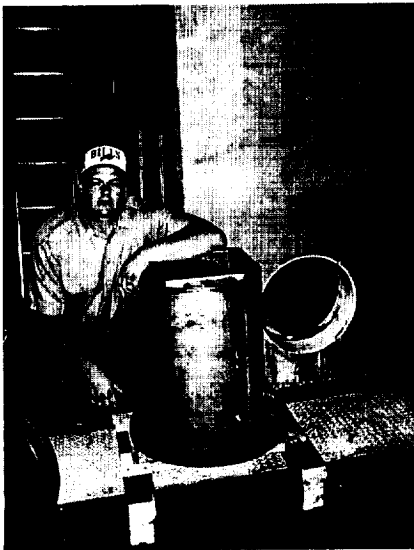
(a) Transition installation.
