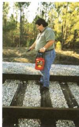
Sun Coast Chemical's Chris Fornili sprays railroad tracks with a special lubricant derived from a lube product developed for NASA's Space Shuttle transporter.
