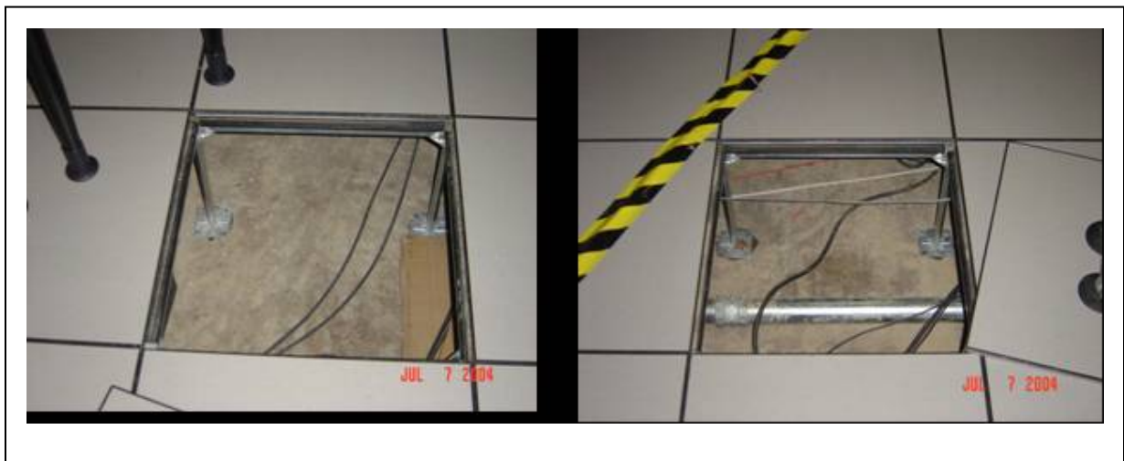
Figure 5b – Below Raised Floor Site
