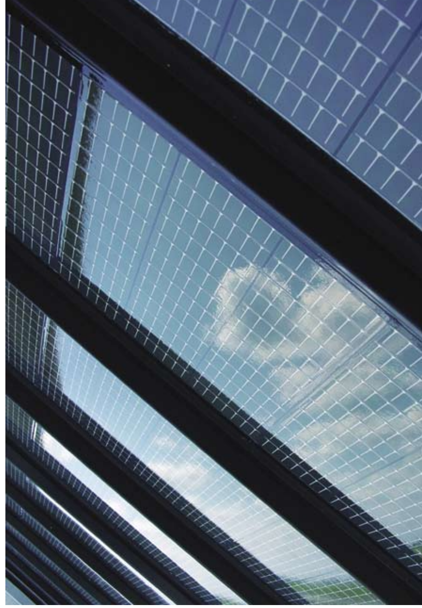
Thin film solar cells derived from amorphous silicon, pictured here, are gaining more and more attention in a market otherwise dominated by mono- and poly-crystalline silicon solar cells.
