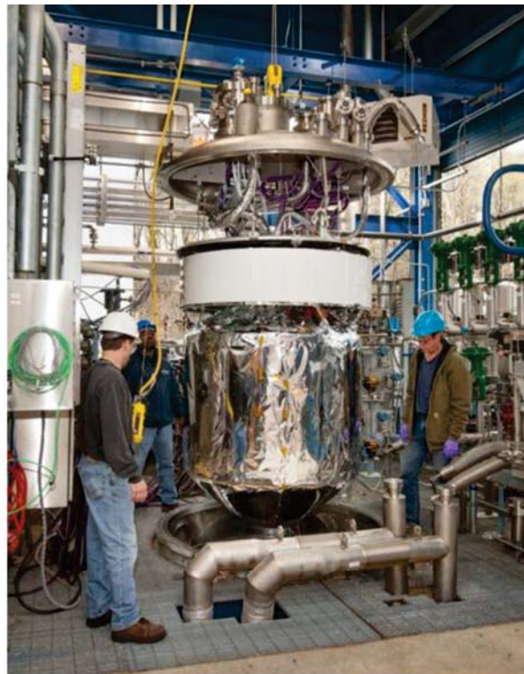
Figure 3. The assembled cryogenic boil-off reduction system test article.
