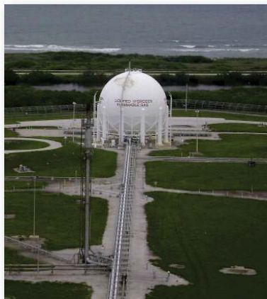
Liquid hydrogen is carried to the launch pad through a cross country line from an 850,000 gallon (3,200,000 L) storage tank. The vertical column is the flare stack where hydrogen boil-off is burned. The Atlantic Ocean is in the background.
