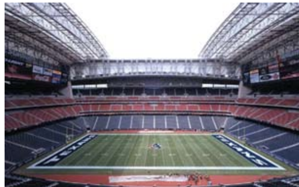
Houston's Reliant Stadium features a retractable, PTFE fiberglass fabric roof crafted by Birdair.
